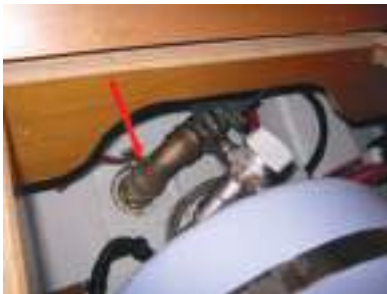
Galley draining + Cool box Saloon seating Starboard
