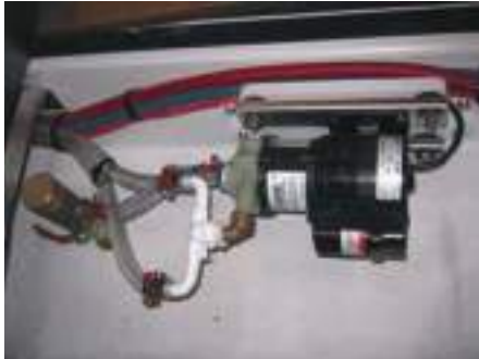
Seawater inlet + Pump
