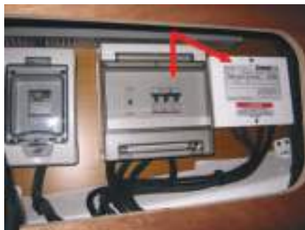
Relay box + Differential (Ref 3)
